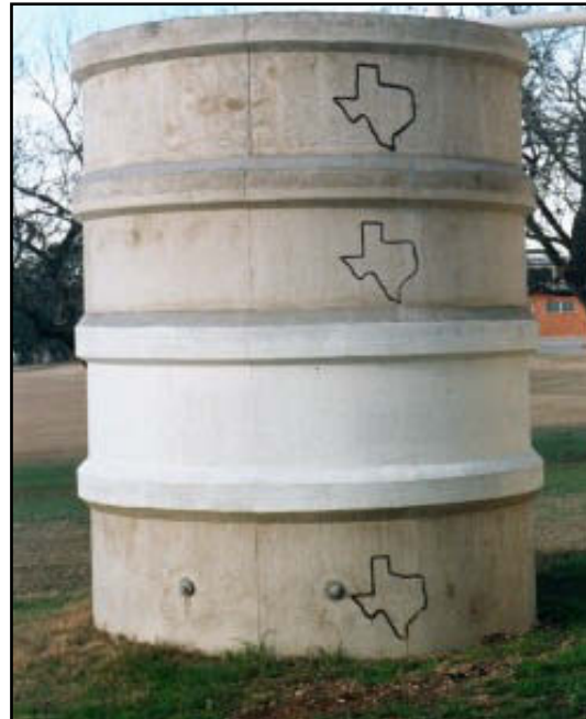
Figure 2-9. Concrete tank fabricated from stacking rings of concrete
